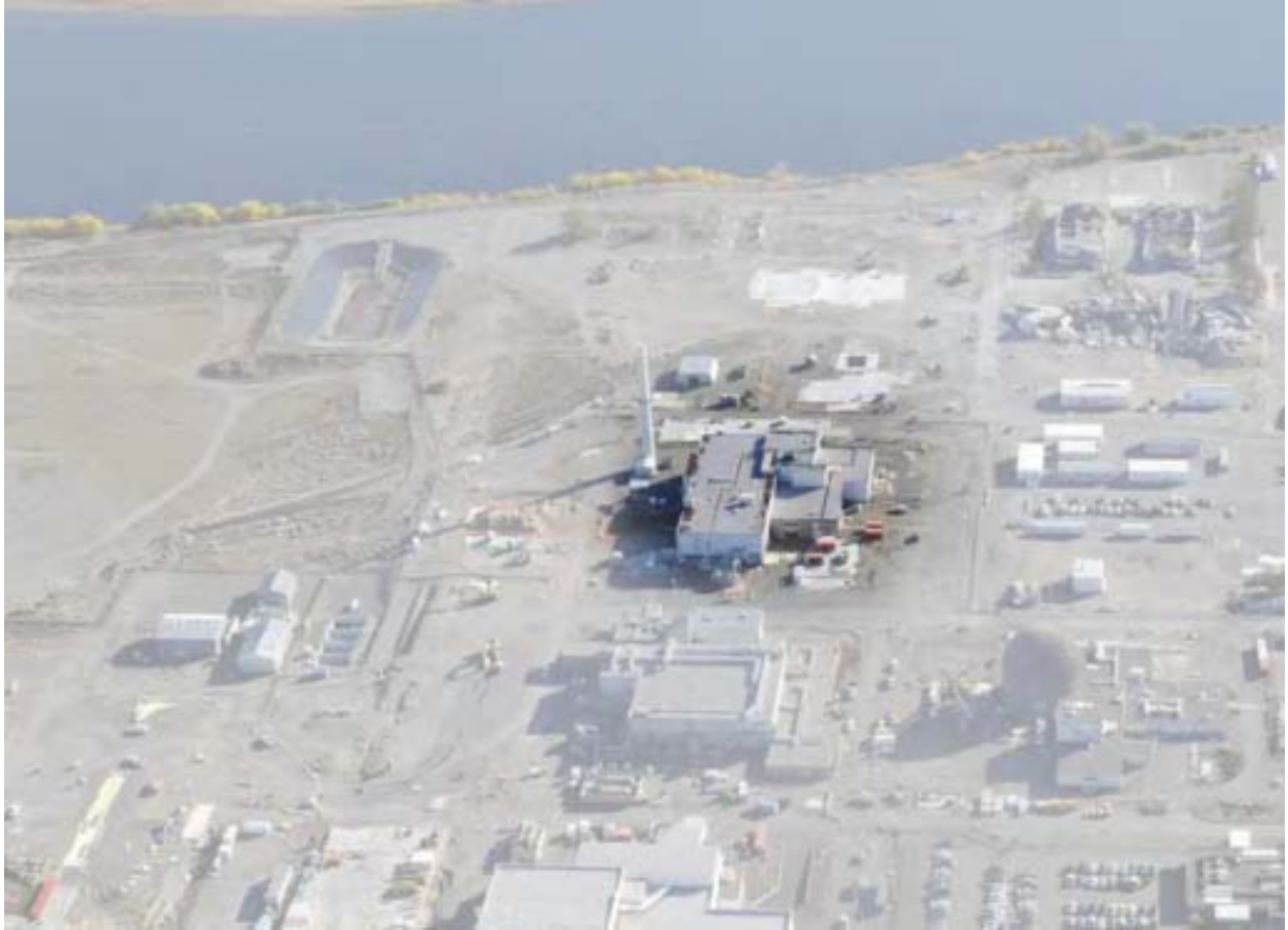
Figure F.2-1. Building 324
